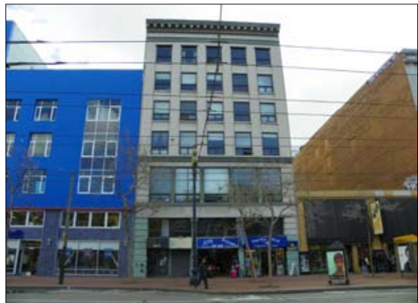
Sterling Furniture Building (1907) Brick with wood posts Source: TKC
